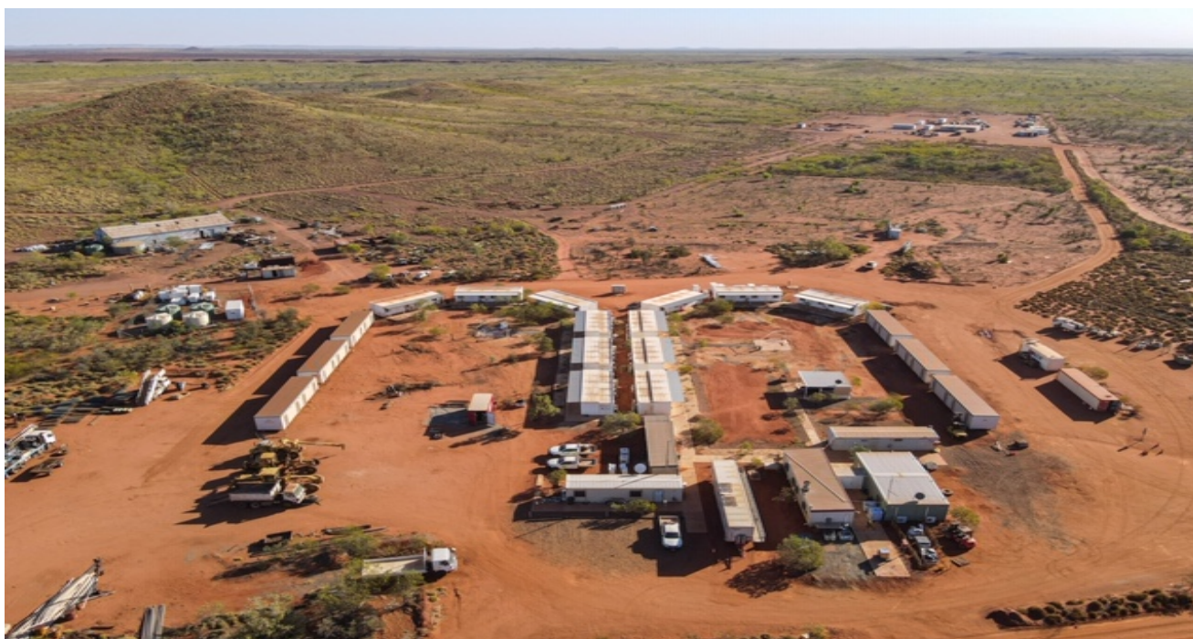
Photo 2: Wingina Camp near Indee Station – Upgrade in Progress
