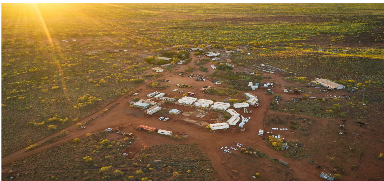
Photo 1: Wingina Camp near Indee Station – Before Commencement of an Upgrade
